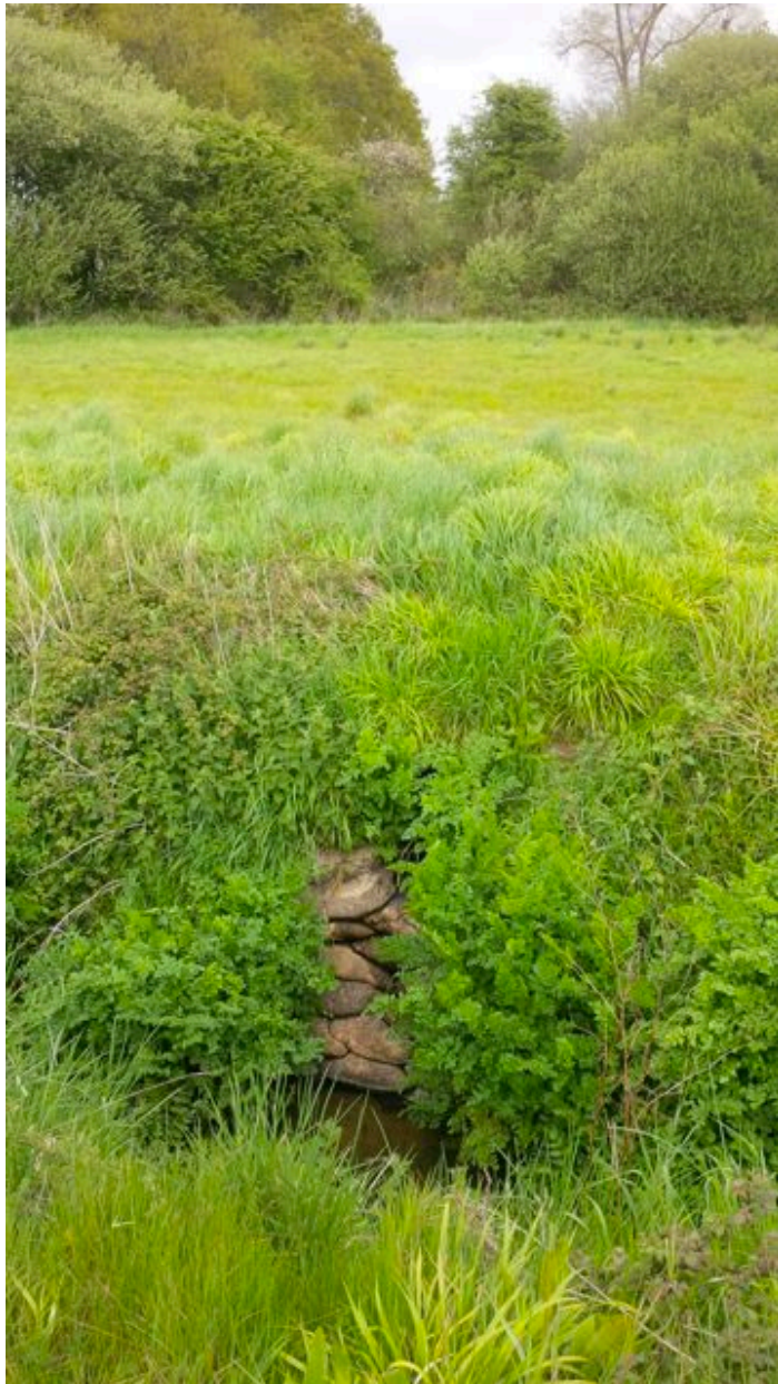
Picture 6 – A culvert connects the pond near the site centre to the wet ditch running along the western boundary.
