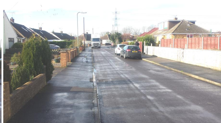
Fig 05. Altern Road – Western view
