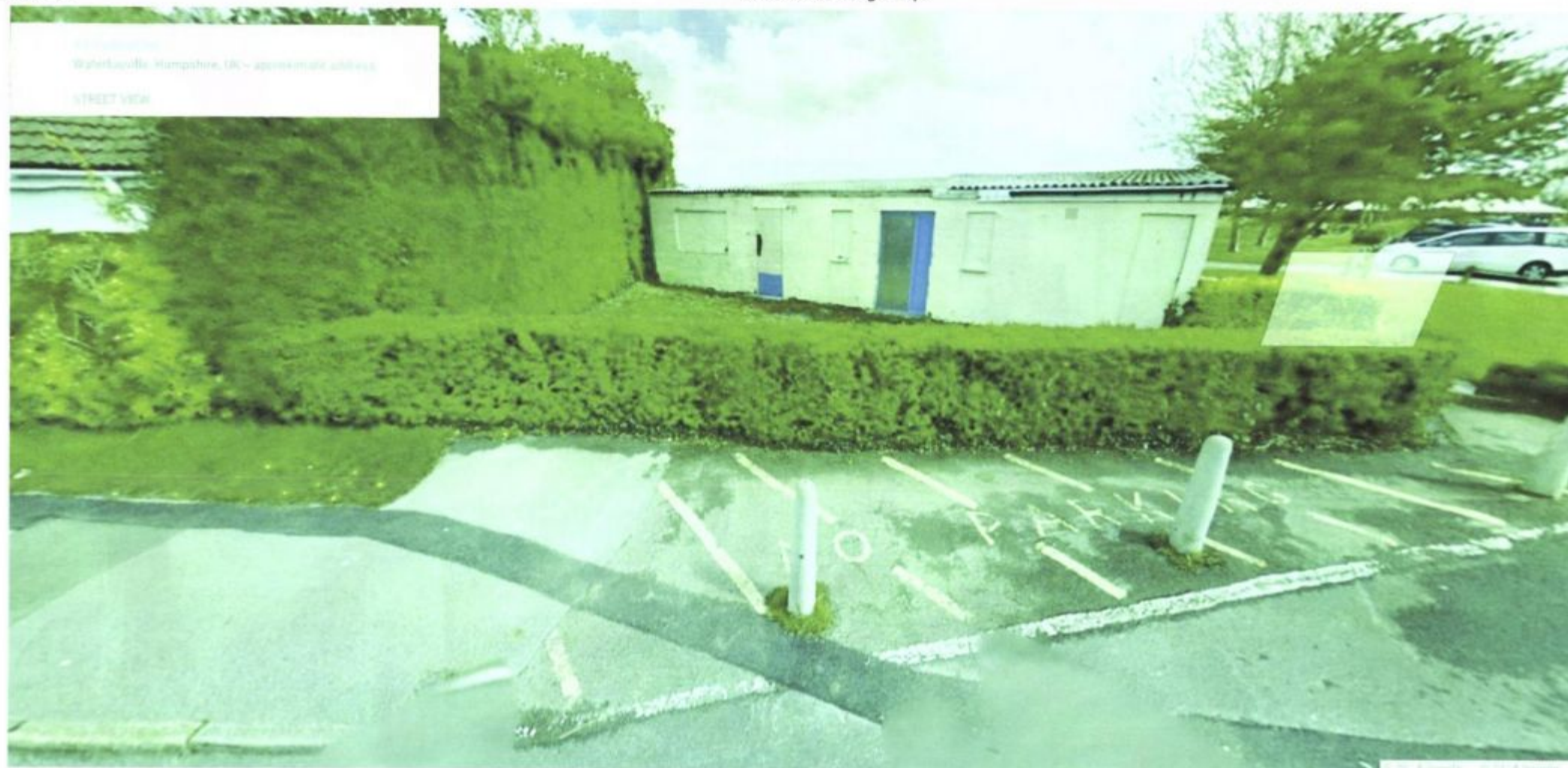
REAR OF PAVILLION
