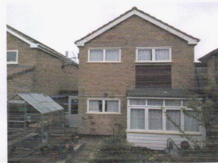
PHOTO REAR ELEVATION
