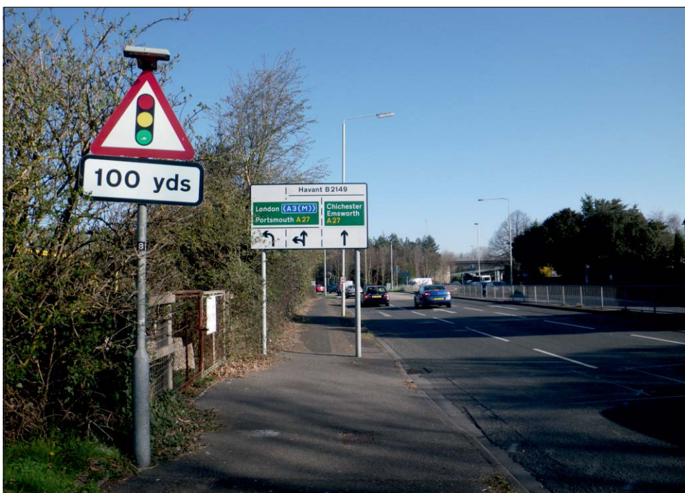
Plate 1: North facing shot of eastern Site boundary showing A3023 carriageway
