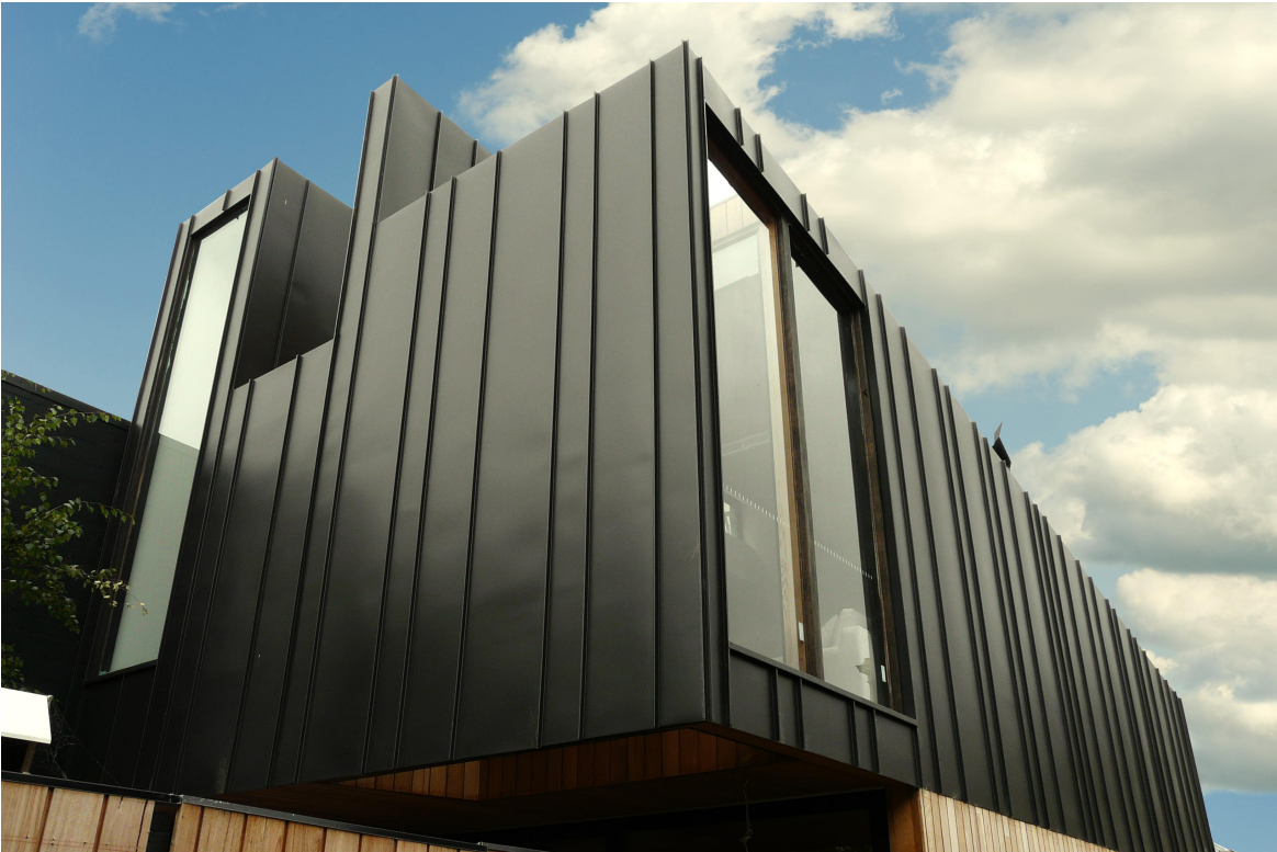
Example of Rheinzink zinc used on a vertical element
