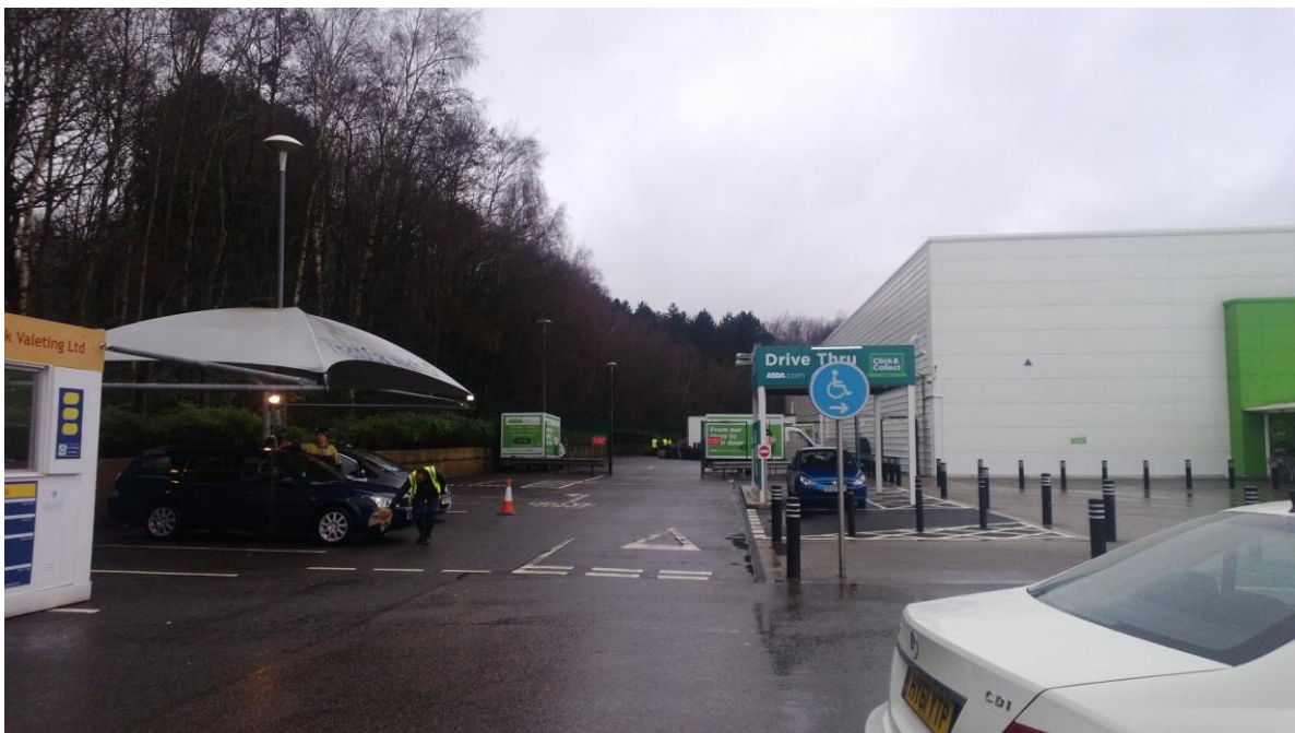
Photo 2. Showing screening of site
