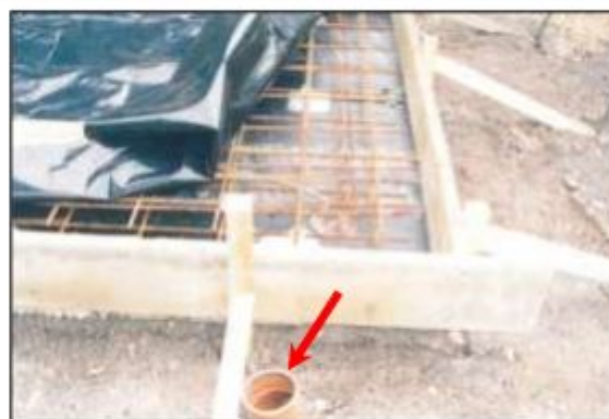
Photo 43: This reinforced base slab for a double garage has drainage provision (red arrow) beneath the structure to redirect roof runoff to supply roots with water.
