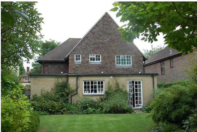
Current rear of property displays flat roof extension.
