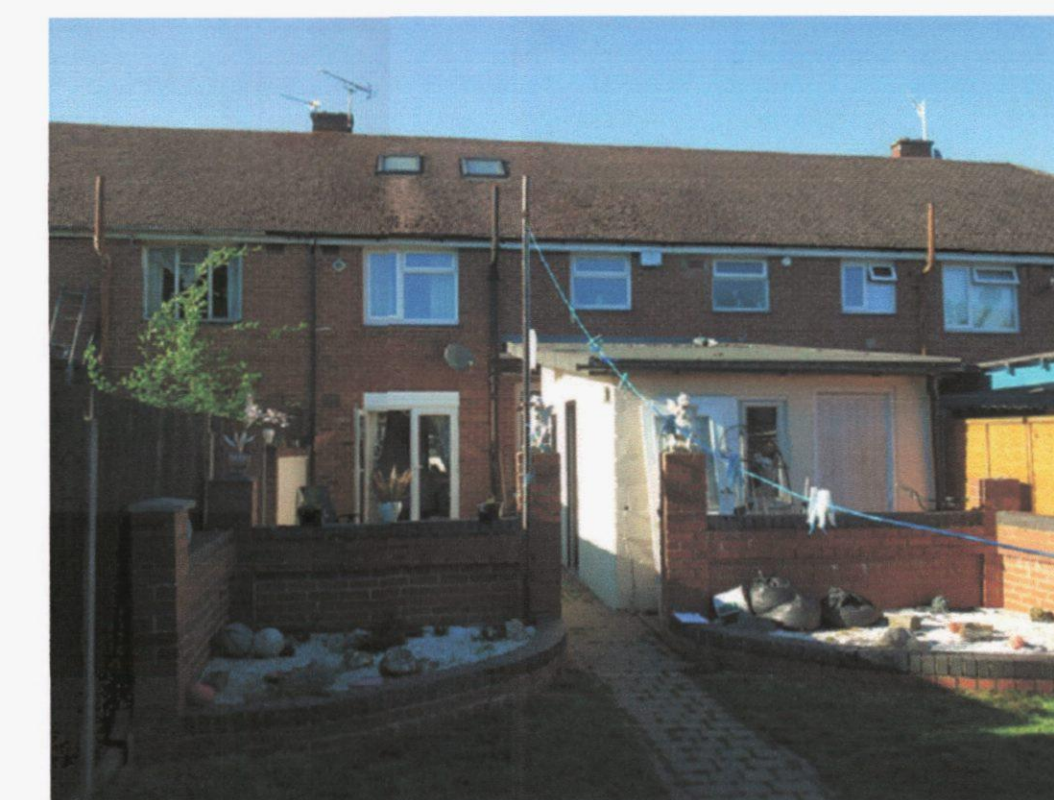
PHOTO REAR ELEVATION
