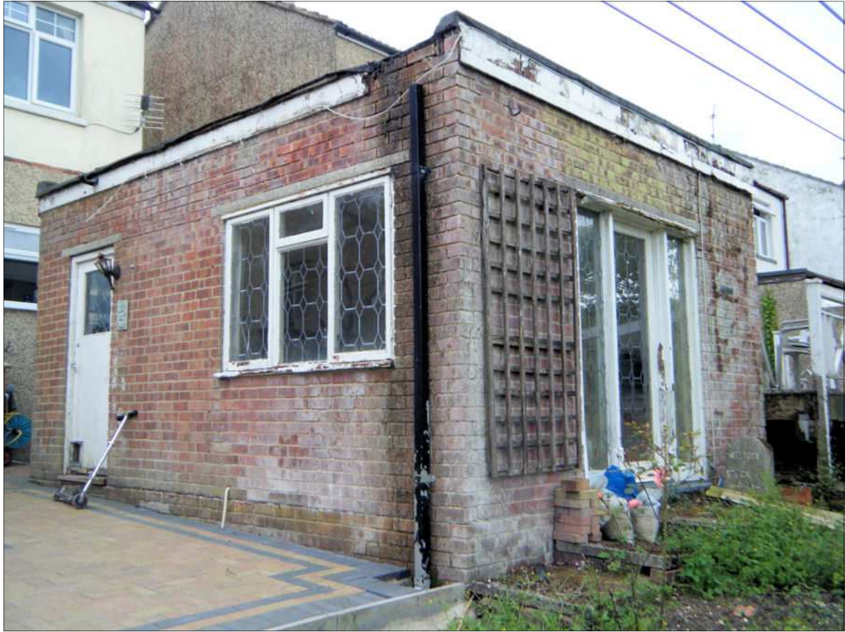
Rear and side view of workshop.
