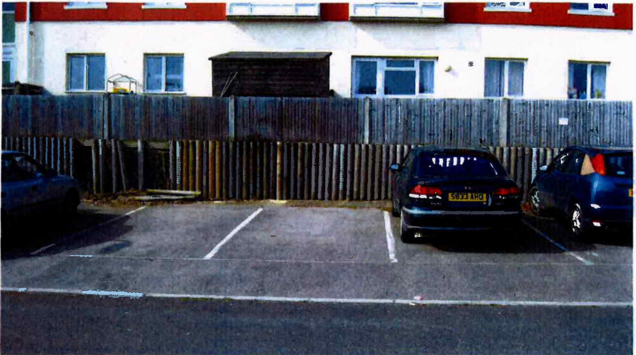
Photograph A – View of retaining wall with highway and parking areas in the foreground and properties in the background.
