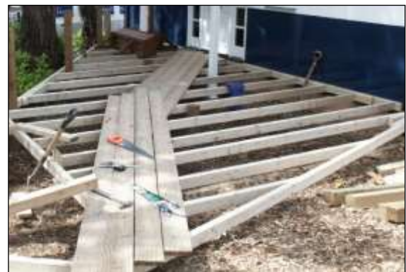
Photo 35: This deck supported above the ground on small posts provides a low-impact alternative to conventional patio surfacing in RPAs.
