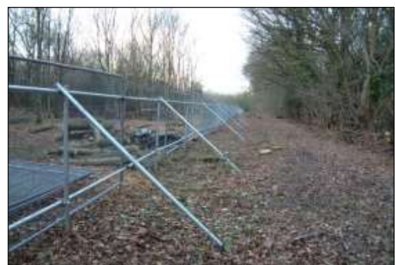
Photo 2: Heras fencing wired to scaffold braced posts is a
