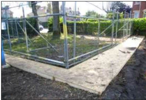
Photo 9: Plywood fixed to a wood frame is another effective method of protecting soil from pedestrian compaction.
