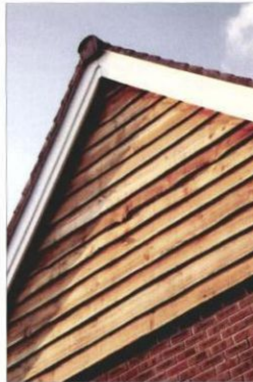
Photo 4 : Wavy edge boarding on garages
