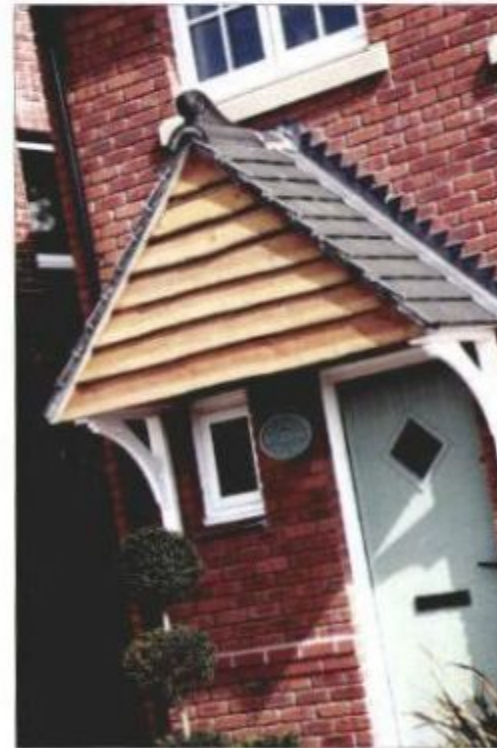
Photo 5 : Wavy edge boarding on porches
