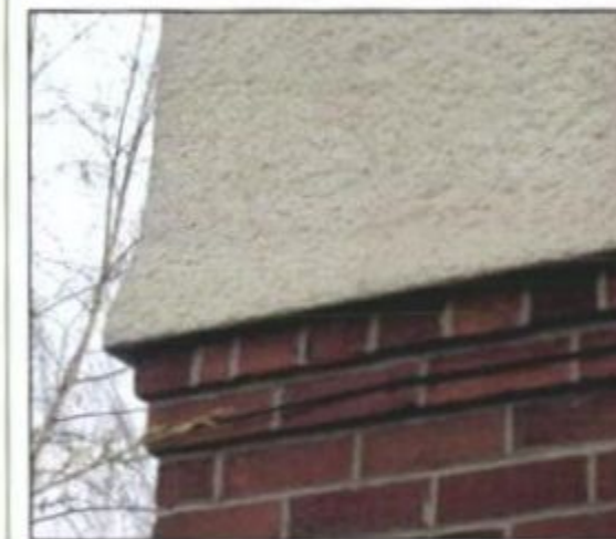
Photo 8 : Render to brick bellmouth detail on Arts and Crafts cottages at Greenhill Road, Winchester
