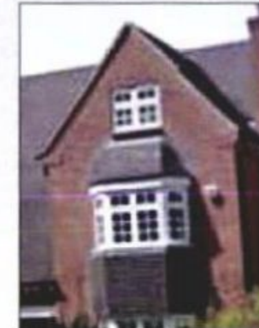
Example of darker roof tile also being used for tile hanging to double height bay
