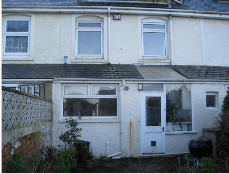
(image showing existing)
