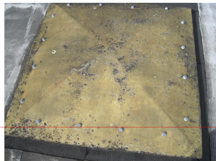
EXTERNAL VIEWS OF ROOFLIGHTS SHOWING PERISHED CONDITIONS.
