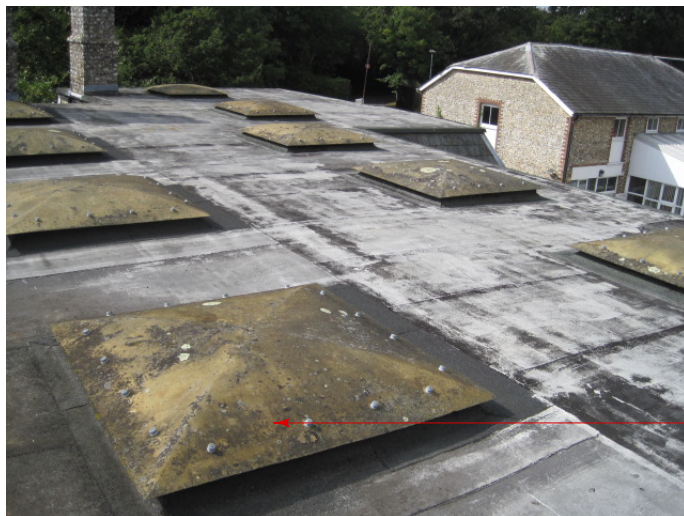
EXTERNAL VIEWS OF ROOFLIGHTS SHOWING PERISHED CONDITIONS.
