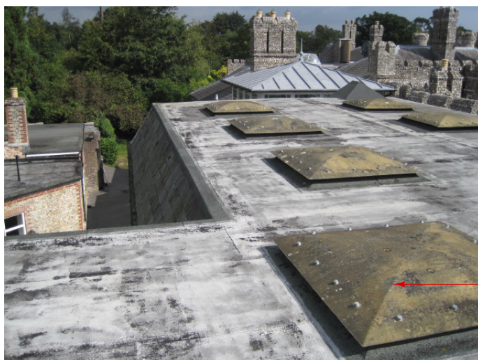
EXTERNAL VIEWS OF ROOFLIGHTS SHOWING PERISHED CONDITIONS.
