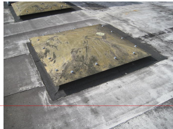
EXTERNAL VIEWS OF ROOFLIGHTS SHOWING PERISHED CONDITIONS.
