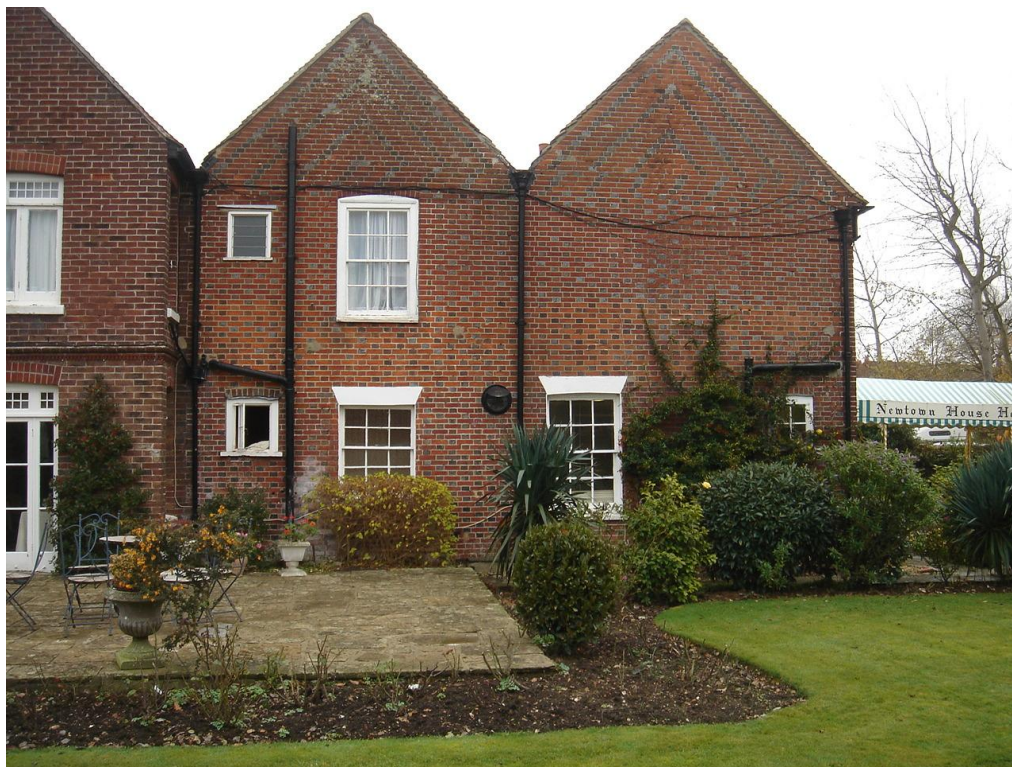
2.2 Terrace and adjoining windows to office and WCs.
