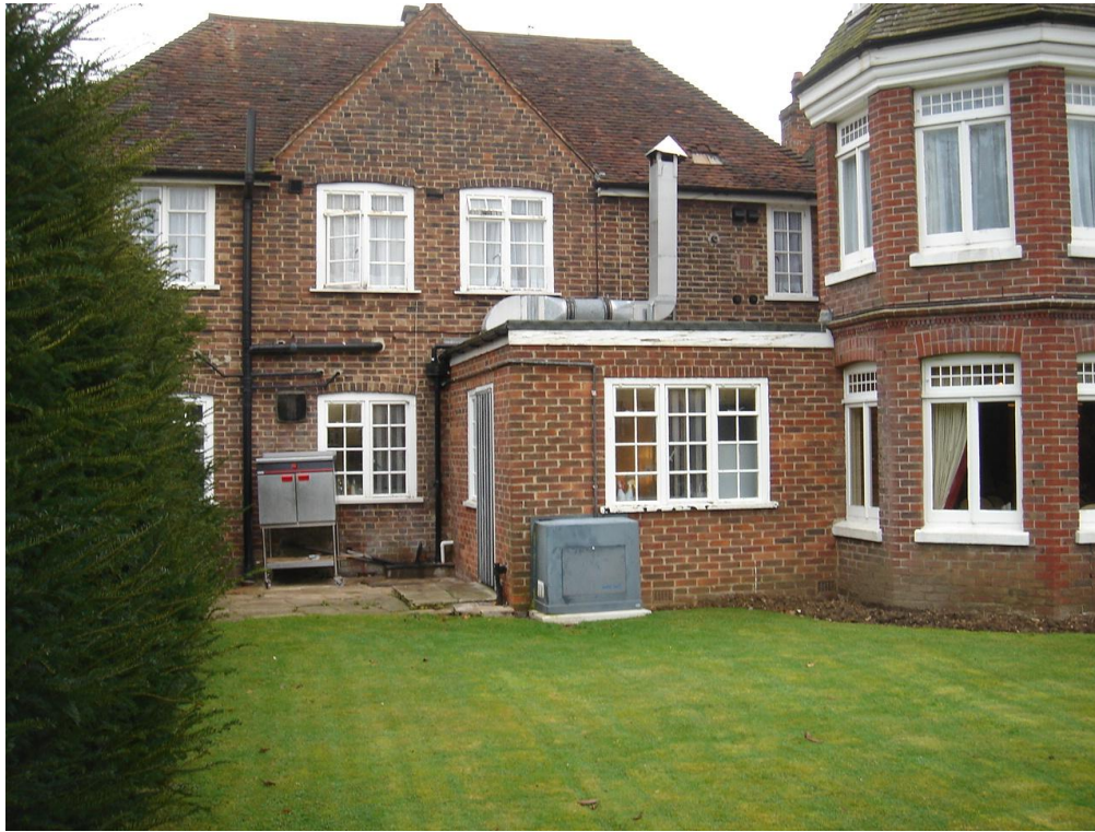
2.4 Kitchen area adjacent to restaurant
