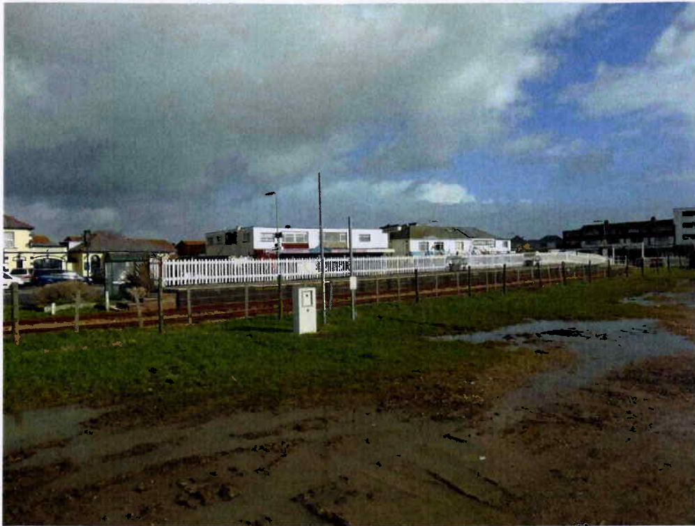
Image 3: Existing South elevation of the site at Eastoke Corner.
