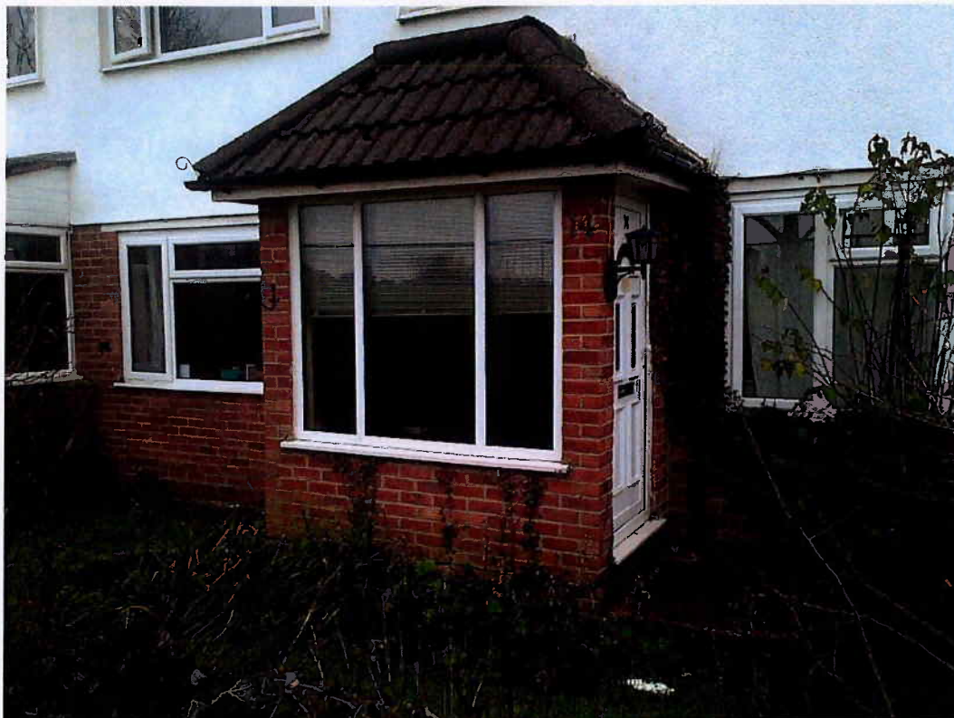
2. View to front of house showing porch
