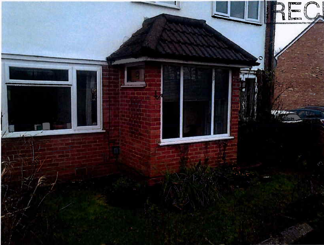
1. View to front of house showing porch
