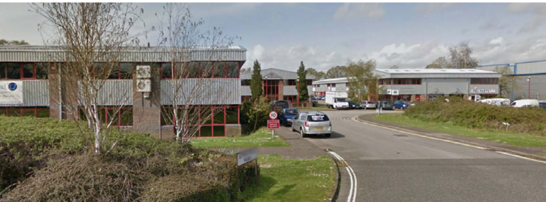
View along Elettra Avenue of industrial units
