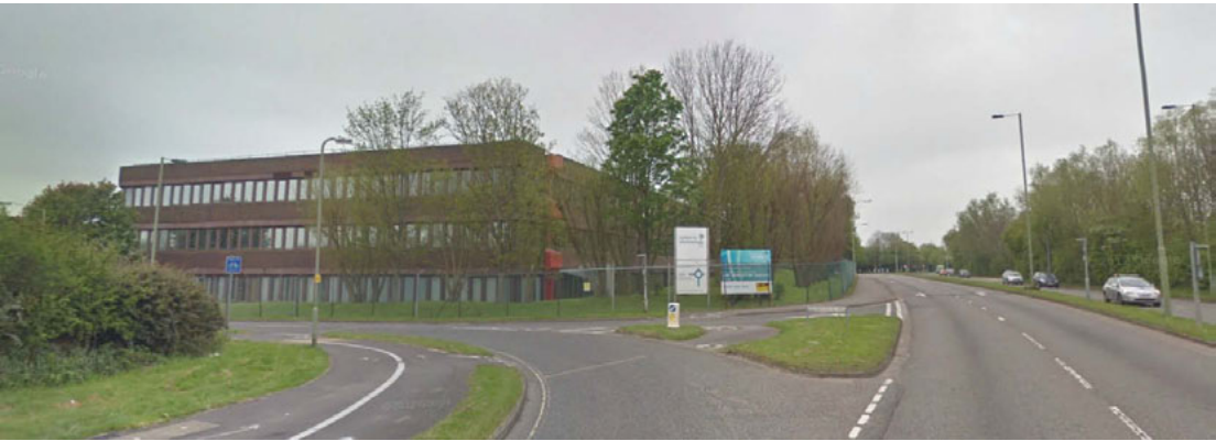
View along Hambledon Road of existing 3-storey office building
