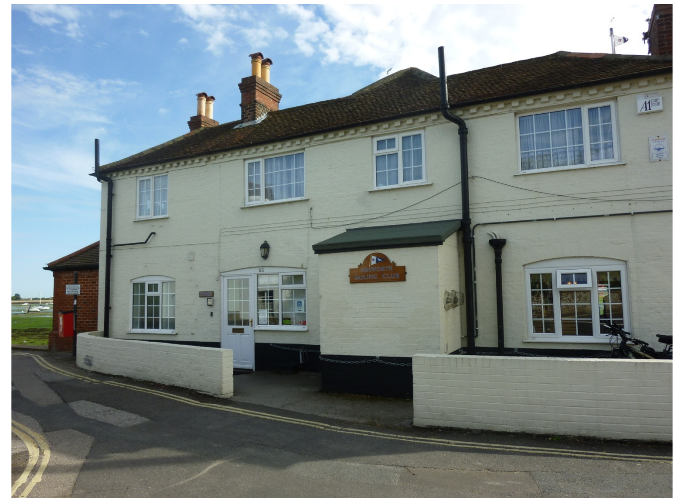
North elevation – Photo from 2011 prior to fire and re-painting
