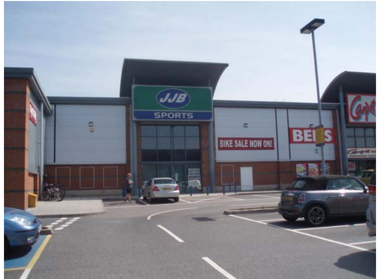
Photo of Existing Front Entrance Elevation
