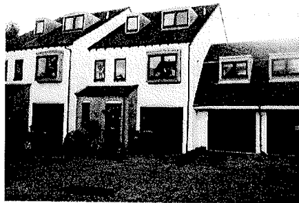
Fig 1 – Front view of the property within courtyard
