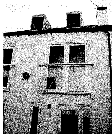
Fig 2 – Rear view of the property within garden.
