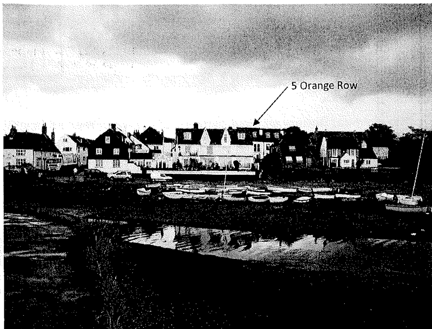
Fig 4 – View of property from millpond footpath
