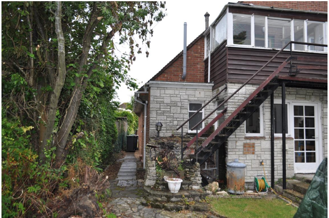
(View of south elevation showing boundary between No.30 and No.28.)
