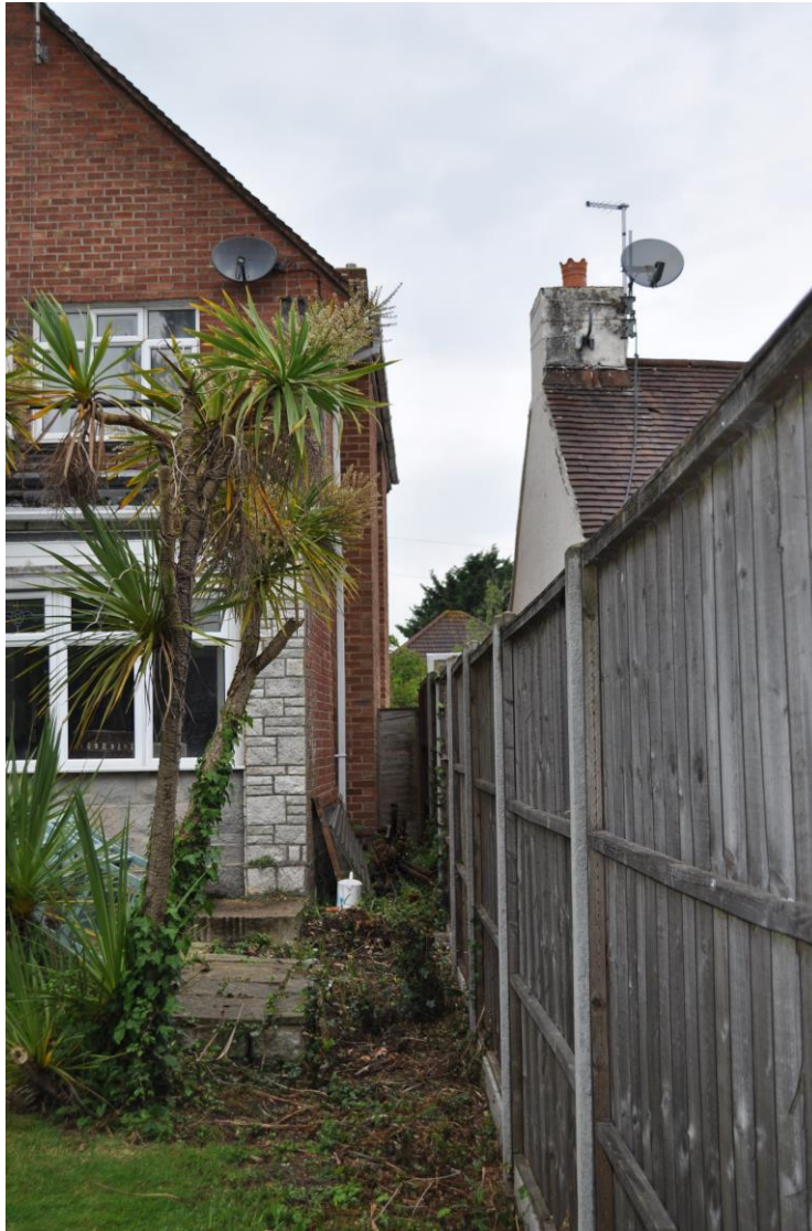
(View of south elevation showing boundary between No.30 and No.32)
