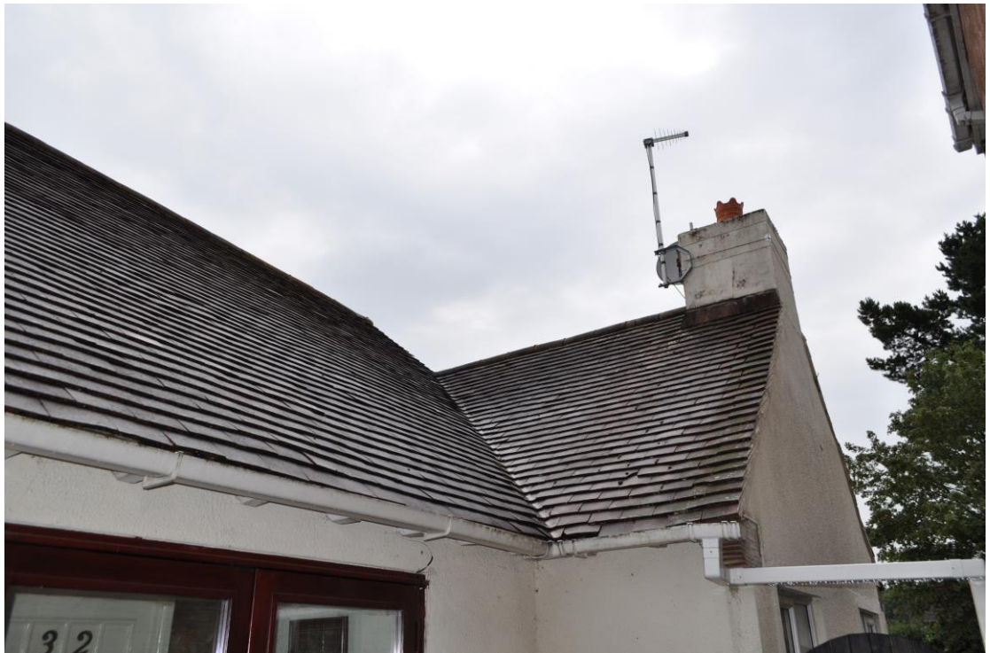
(View showing roof and gable structure of No.32 that proposed side windows would look onto.)
