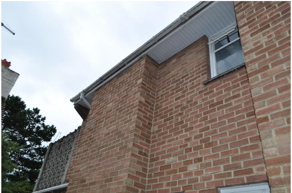
(Current east elevation showing existing side windows)
