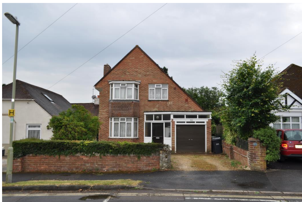
(North elevation of No.30 Warfield Crescent in context with No's 28 and 32.)
