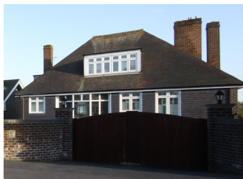
No. 41a with slate tile hanging and slate roof
