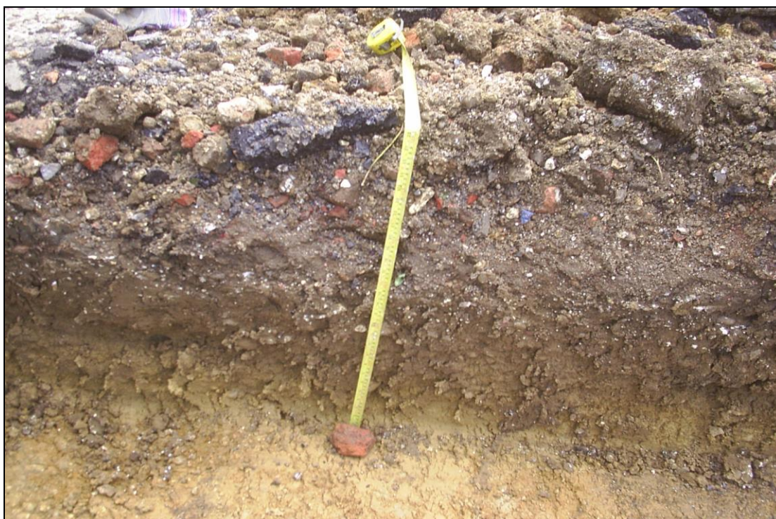
Photograph 10 Showing the ground conditions during preliminary excavations
