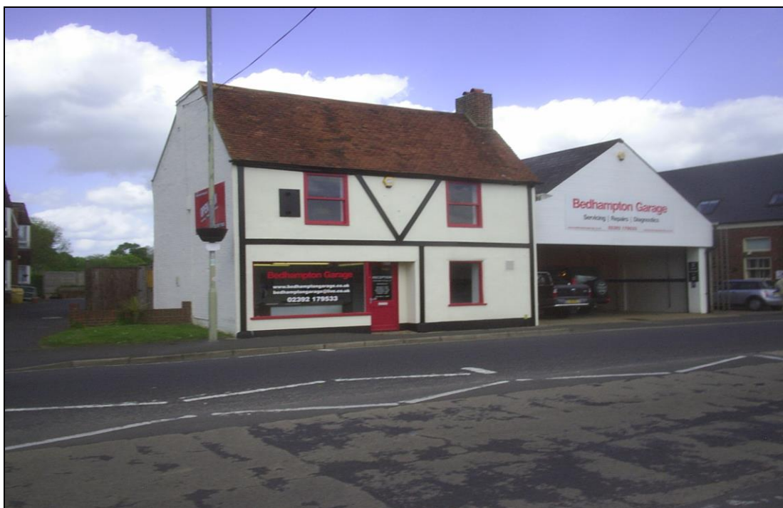
Photograph 7 Showing Bedhampton Garage to the northeast
