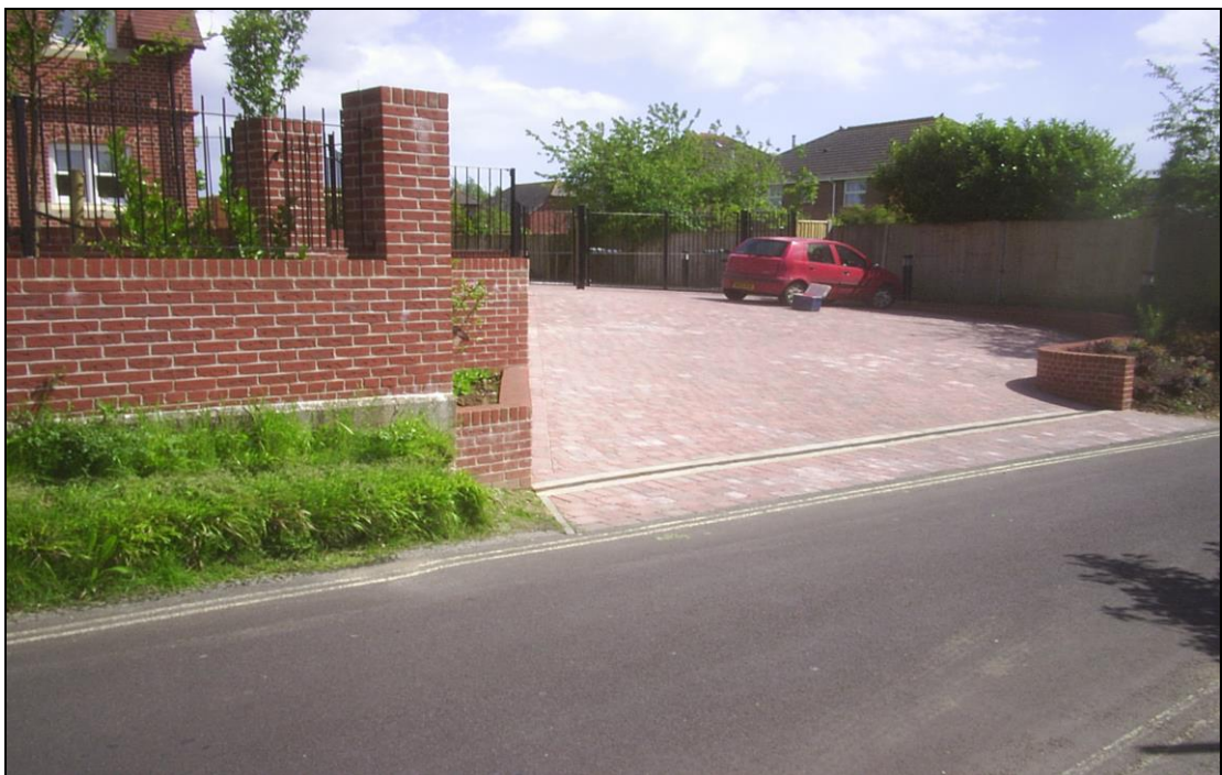
Photograph 9 Showing the ground slope at the rear
