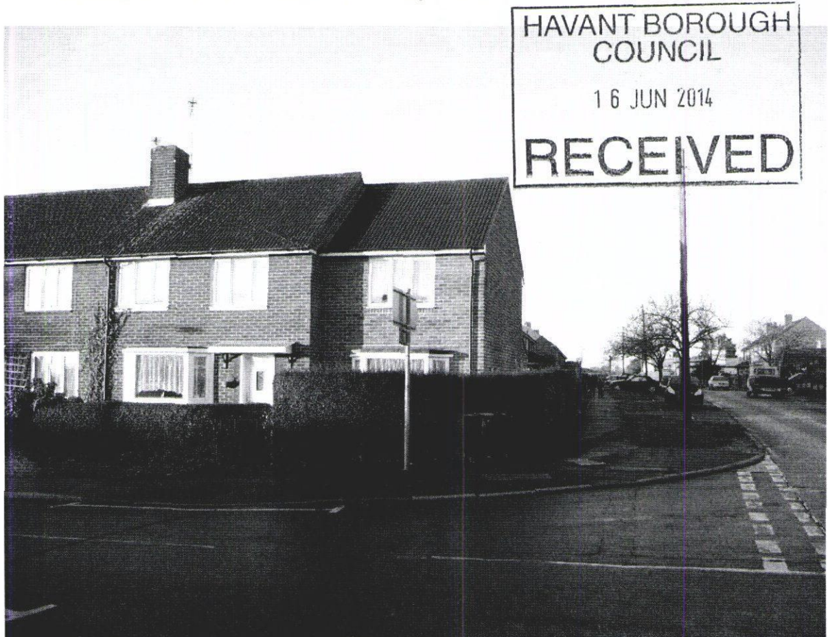
New dwelling at 2 James Road, Havant
