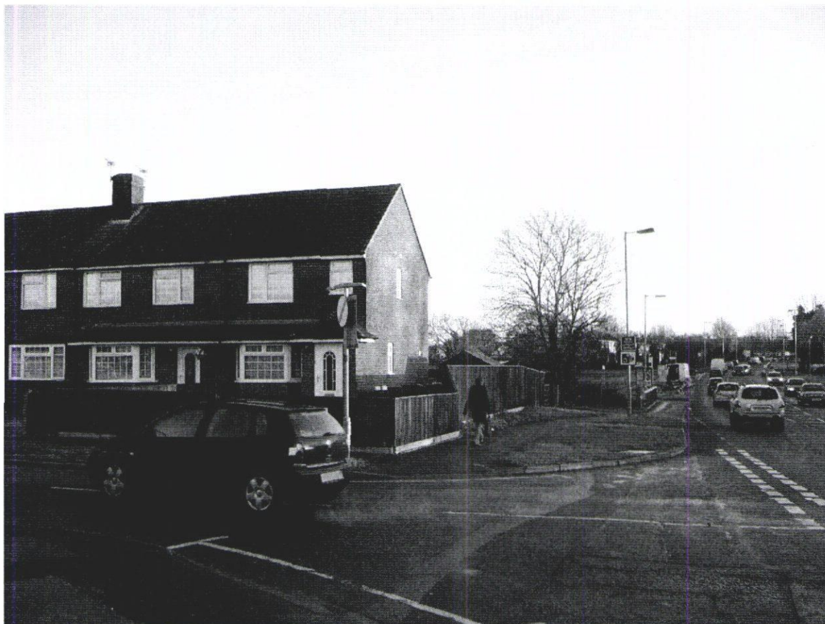
New dwelling at 25 James Road, Havant
