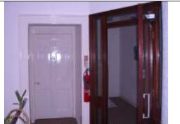
6- The modern addition internal partition wall which is to be removed.
