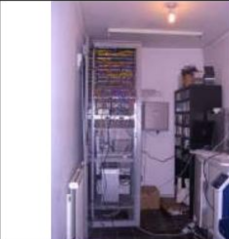
The existing server room to be reinstated as a family bathroom once again.
