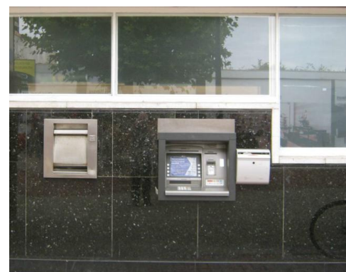
EXISTING ATM WALL
