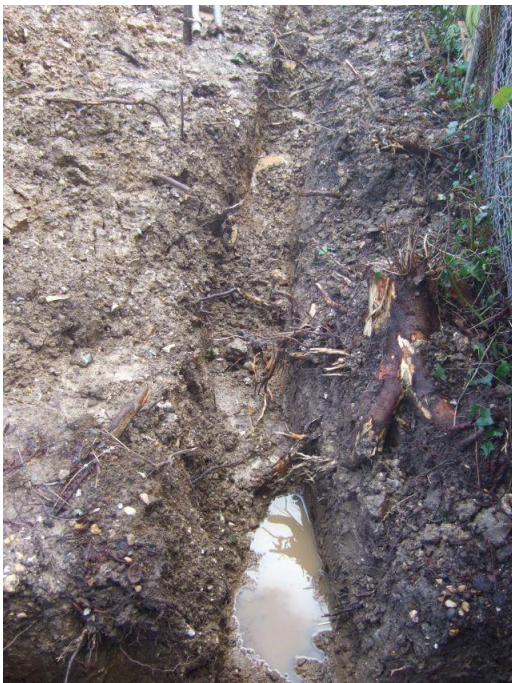
Trench B - Only roots evident from old Sycamore stump
