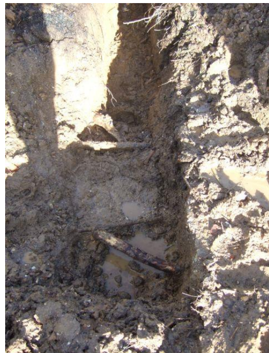
Trench D showing two roots 60mm diameter
