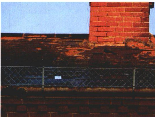
Gaps in roof of rear extension
