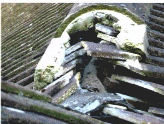
Gaps in roof of rear extension
