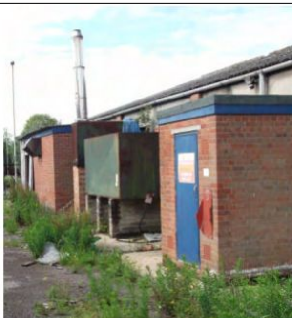
Photograph Four – Flammable liquids store, fuel tanks and boiler room located along eastern site of Unit 25d
