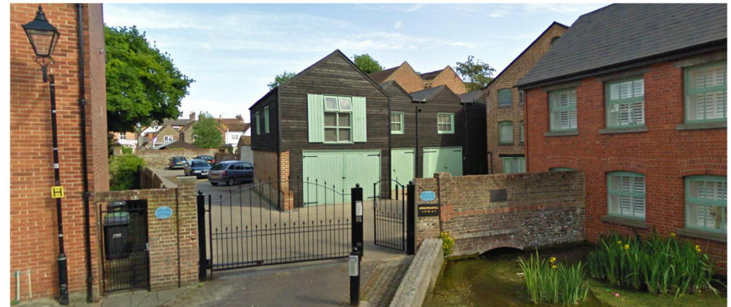
Image 12: Black timber cladding of Springwell development in Havant town centre (courtesy of google maps 2014)
