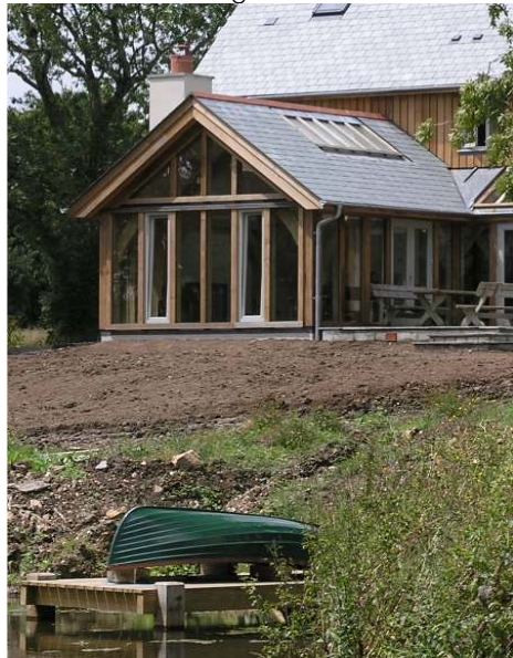
13. Typical barn room, with slate roof
