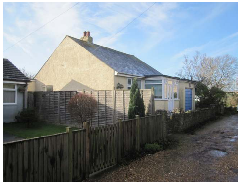
5. View of adjacent property – No. 139, Havant Road.
