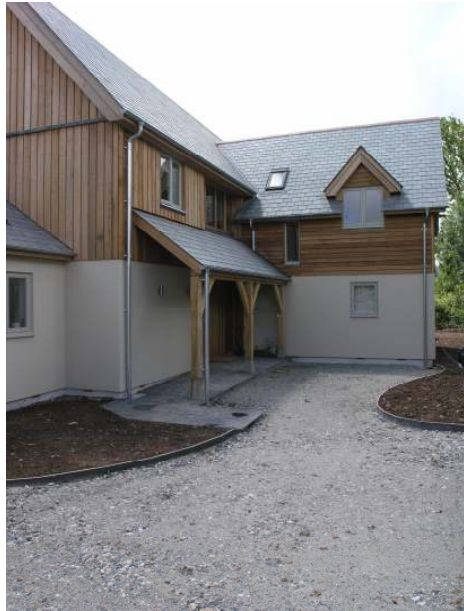
12. Natural slate roof, render plinth & vertical timber boarding.
