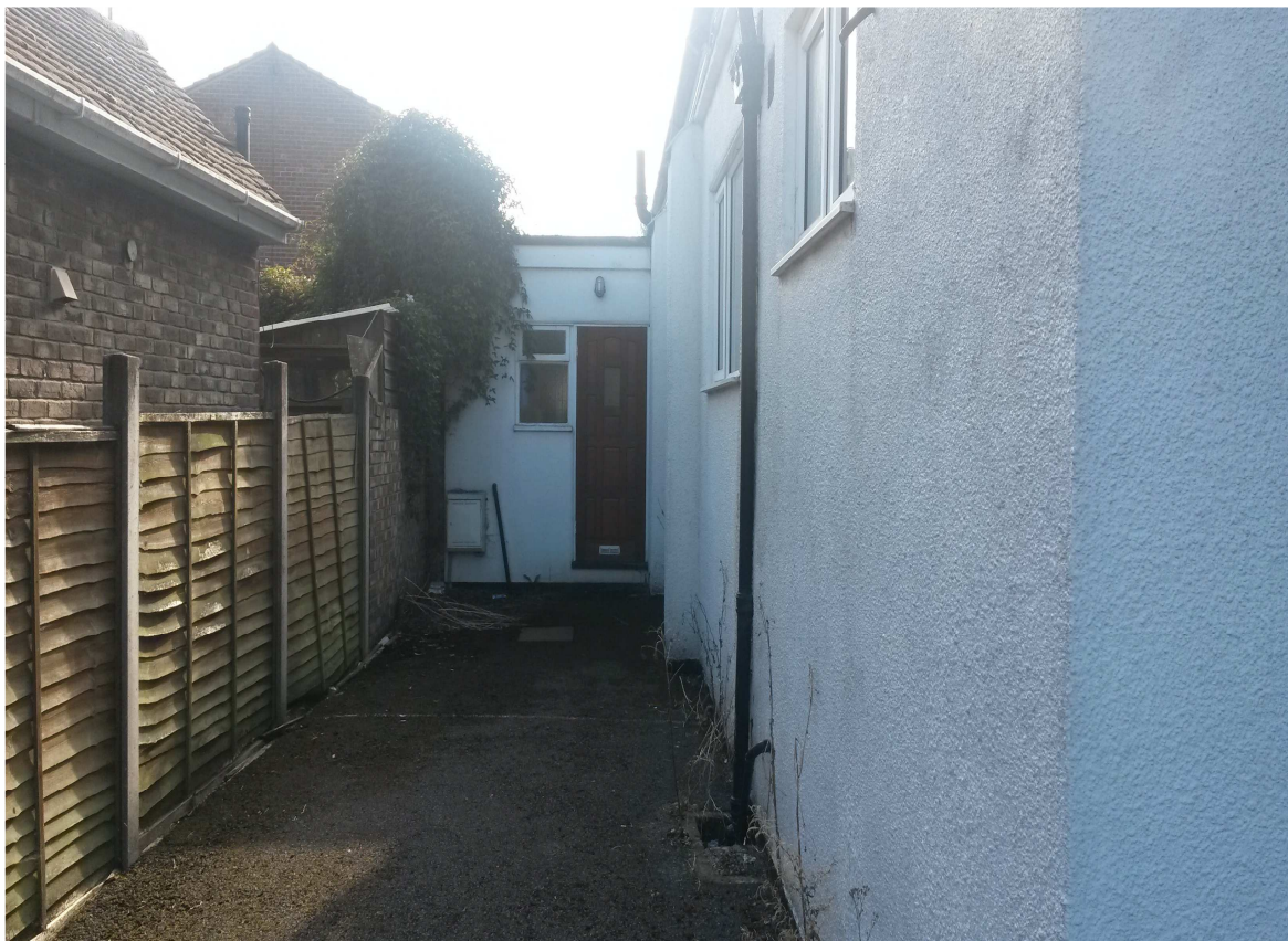
View of east elevation
