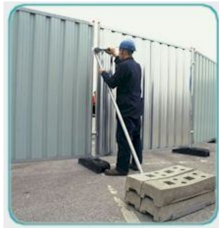
Figure 1: Galvanised metal hoarding
