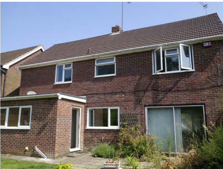
REAR VIEW (SOUTH WEST)
