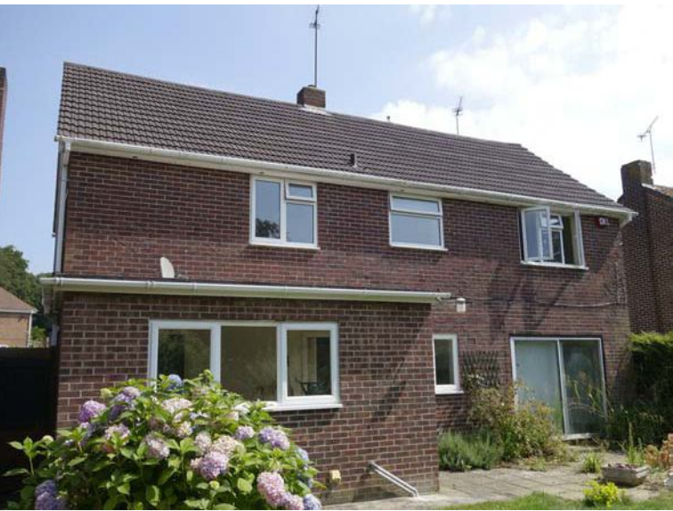
REAR VIEW (SOUTH EAST)
