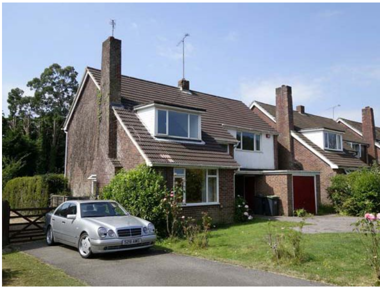
FRONT VIEW (NORTH EAST)
