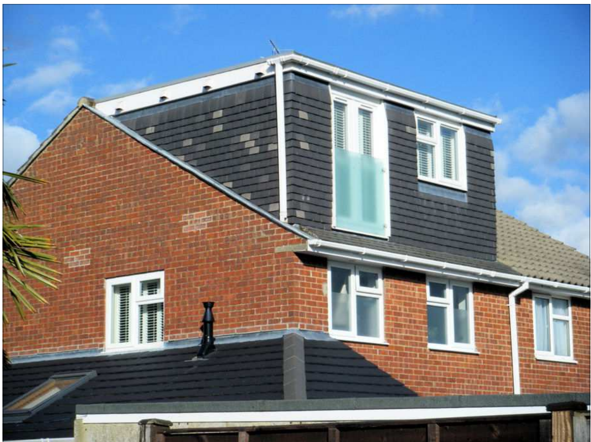
Rear of No. 20 Bedford Close with large rear dormer
