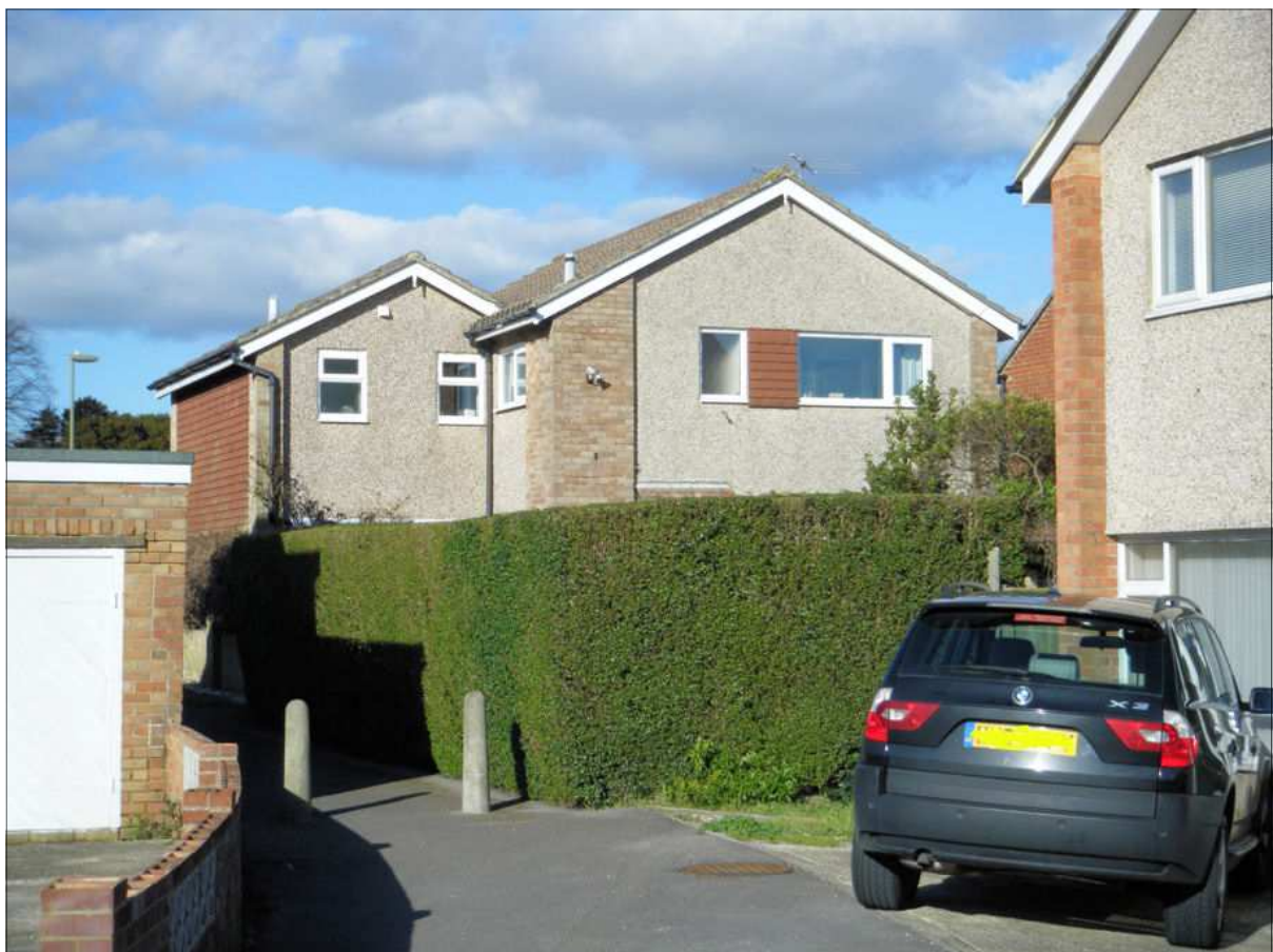
Rear of No. 19 Luard Court with two storey side extension
