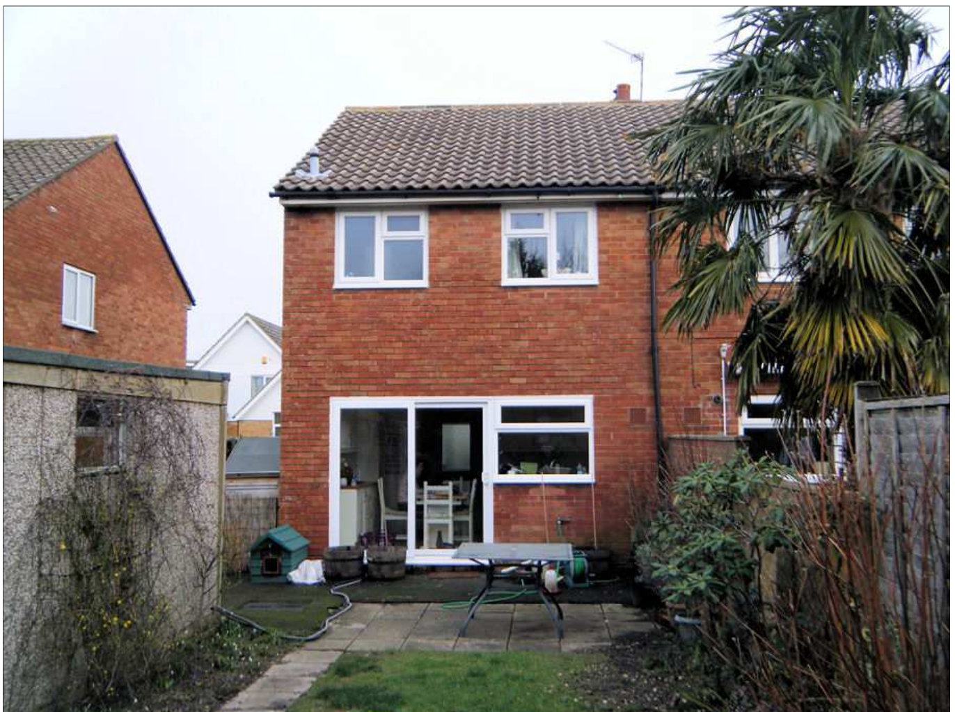
Rear of No. 22 Bedford Close
