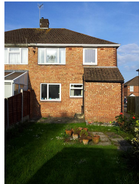
PHOTO REAR ELEVATION
