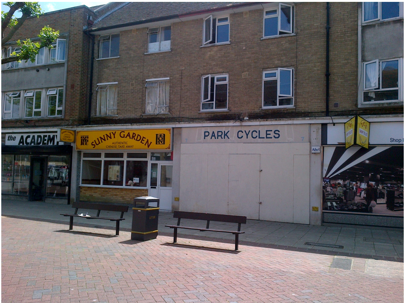
North elevation from Park Parade – shop front currently boarded over.
