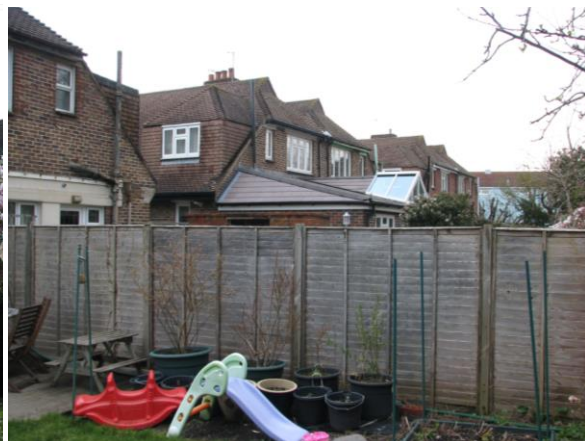
Above: View of Rear of Houses to North
