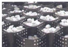
Cellweb TRP access road during filling with clean stone.
