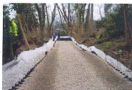
Cellweb TRP access road during filling with clean stone.
