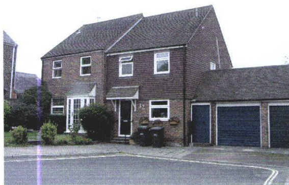
Existing Front Elevation & adjacent property
