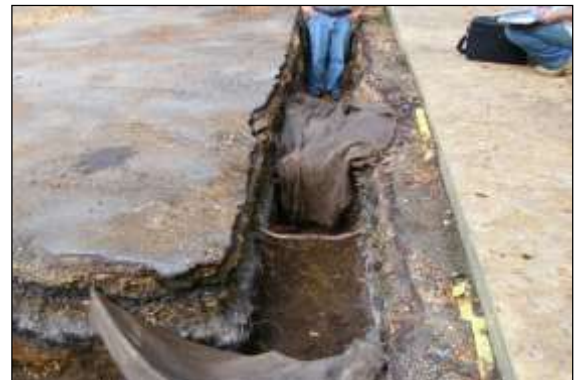
Photo 4: Exposed roots must be protected from light, drying out and extremes of temperature by covering with hessian sacking and boards until they can be covered back with soil.
