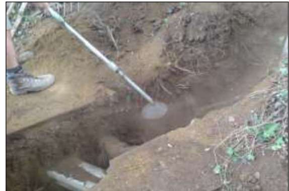
Photo 2: Air spades are very effective at exposing roots and services with minimal damage.
