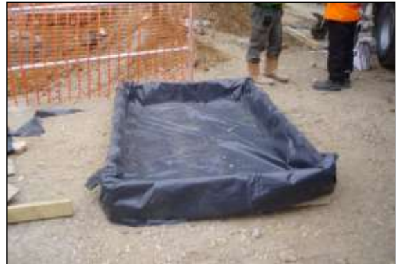
Photo 10: Soil bunding or a supporting framework covered in heavy-duty plastic sheeting is essential where there is a risk of spillages contaminating RPAs. This specifically applies to cement mixing areas and vehicle washing facilities.
