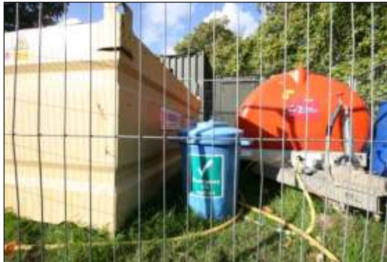
Photo 9: Where fuel or other chemical are stored on site, it is now standard practice to have emergency spillage kits available to restrict the environmental impact of accidents.
