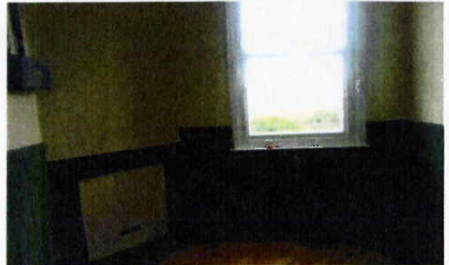
Car park window.
