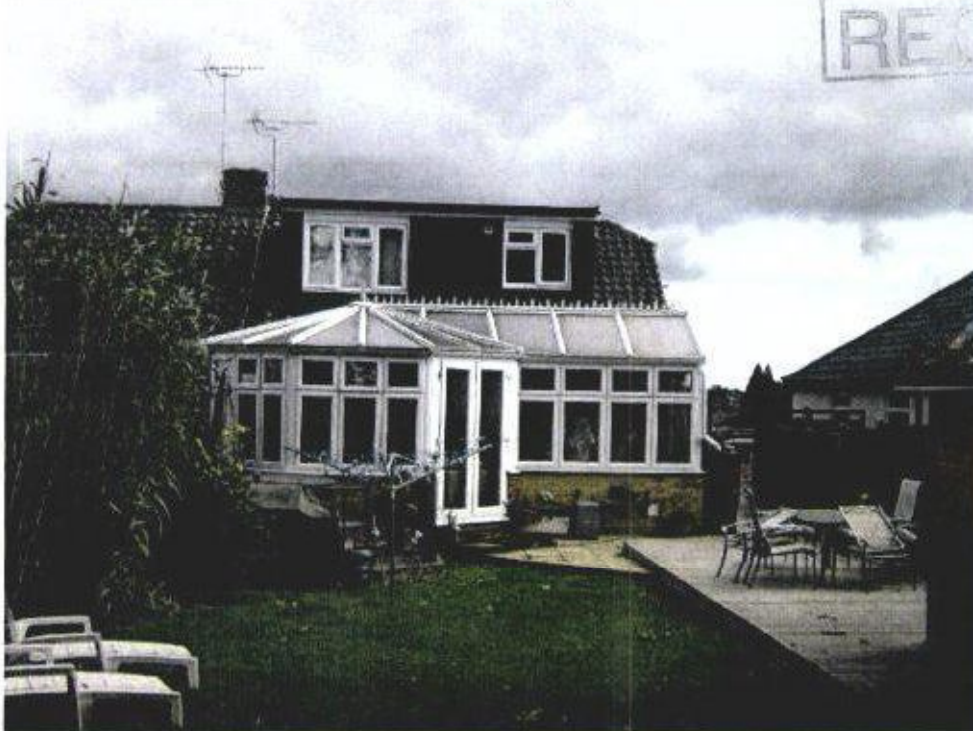
1. View to rear of house and conservatory
