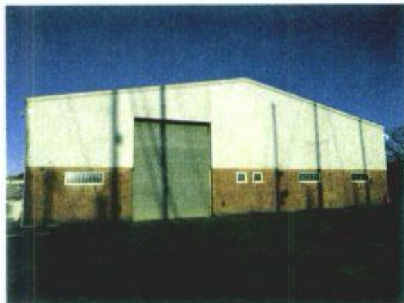
Plate 2: A large warehouse at the centre of the site.
