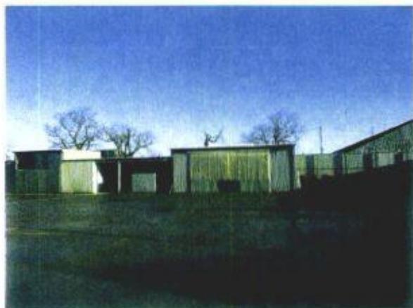
Plate 1: The majority of the application site is hard-standing.
