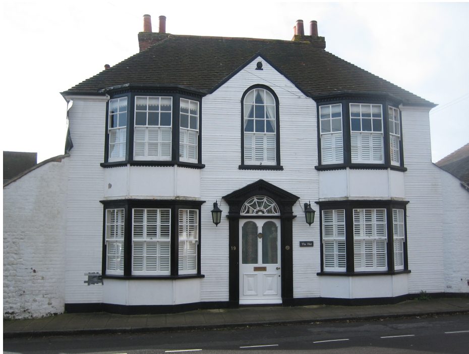
Fig 7 – Principal northern facade of The Hut along King Street.
