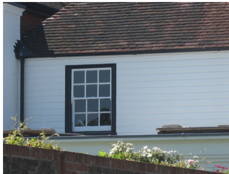
Fig 8 – First floor side window to East elevation
