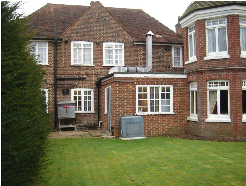
2.4 Kitchen area adjacent to restaurant
