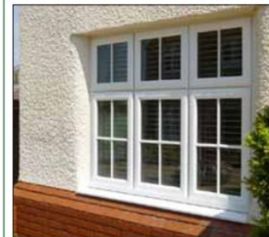
Photo 9 : Roughcast white render rounded into the window reveal
