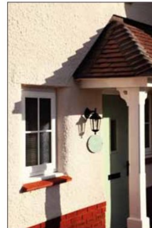
Photo 6: Timber post porch
