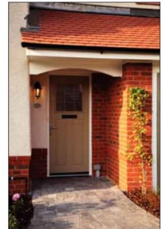
Photo 7: Tile roof porch
