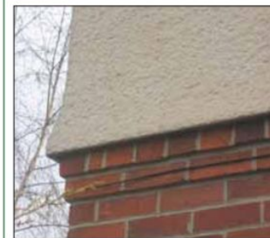
Photo 8 : Render to brick bellmouth detail on Arts and Crafts cottages at Greenhill Road, Winchester
