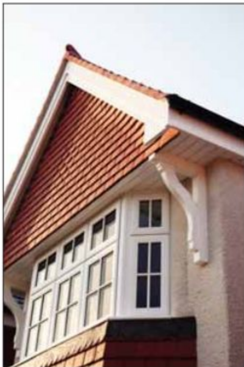
Photo 3: Tile hung gable end
